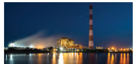
Power from thermal plants - GMR Warora and GMR Kamalanga is
